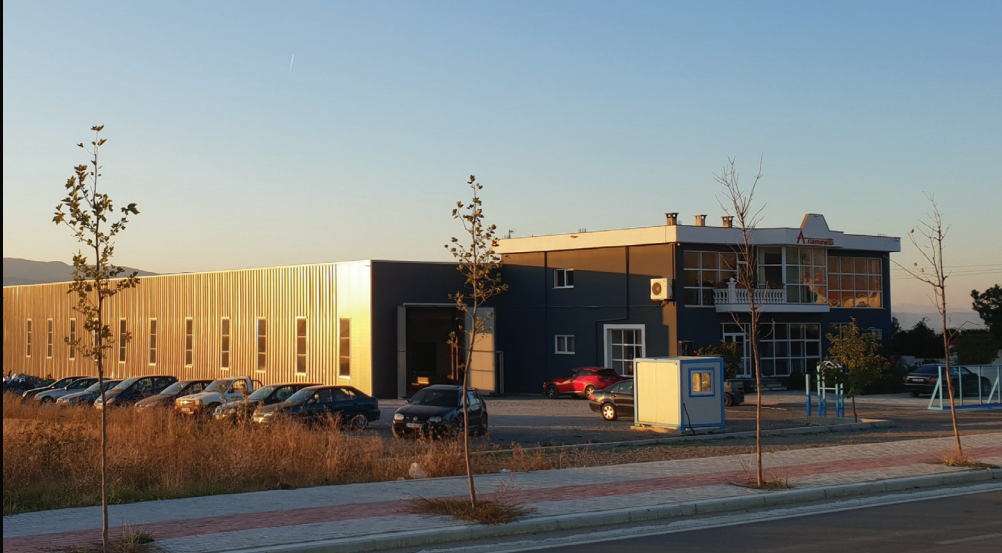
A.caminetti Factory: National road, km 2 Korçë-Ersekë, Albania.
